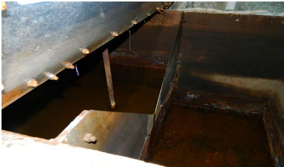
Figure 2: Photograph of Tank TK-C-103 Weir
